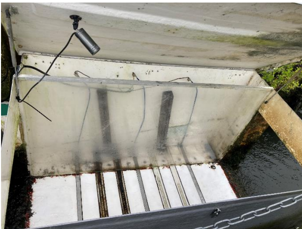
Image 6- This is the fish pass after being cleaned and the new overhead camera having been installed.
