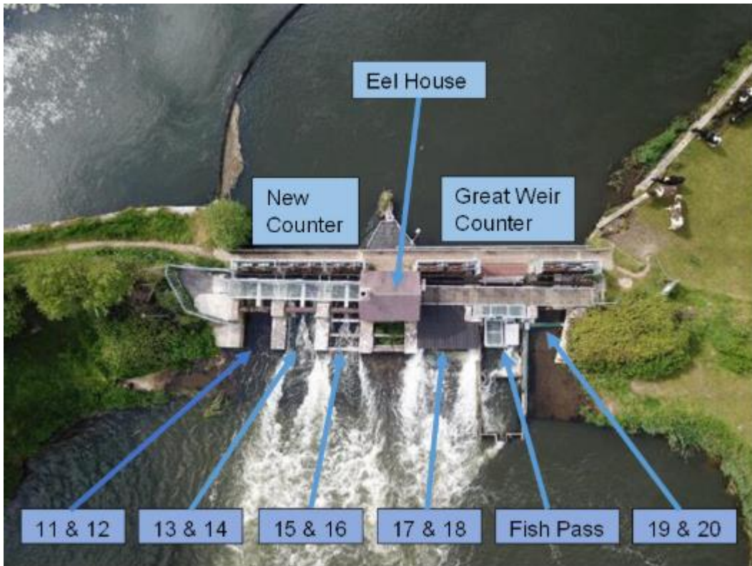
Figure 2 – Labelled image of the Great Weir showing the location of each channel.
